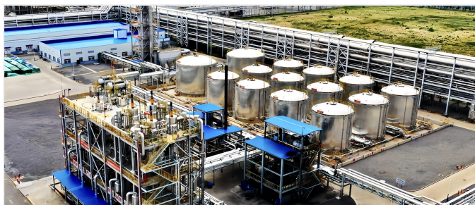
Future Clean Chemicals
